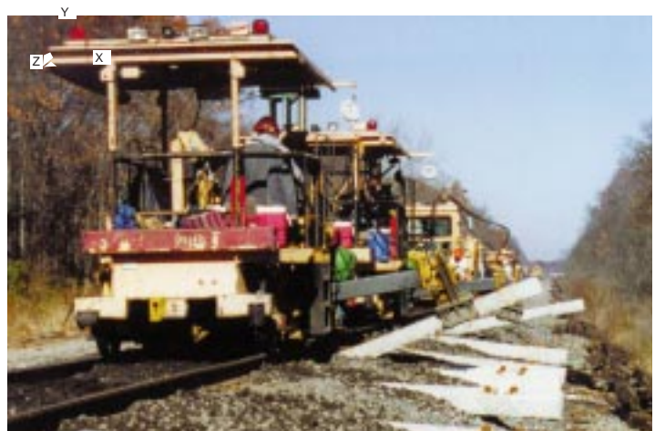
Conventional tie gang installing MRT™.
