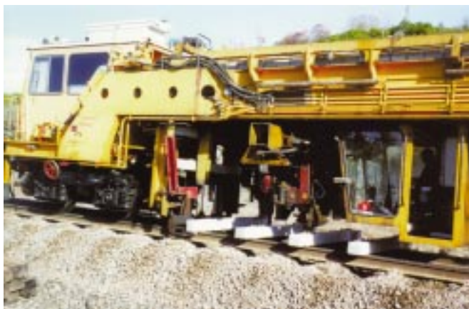
Automated installation with Plasser THS 2000.
